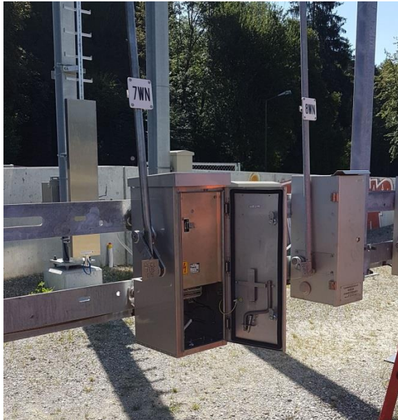
Successful test installation of the MDR3 – motor drive
